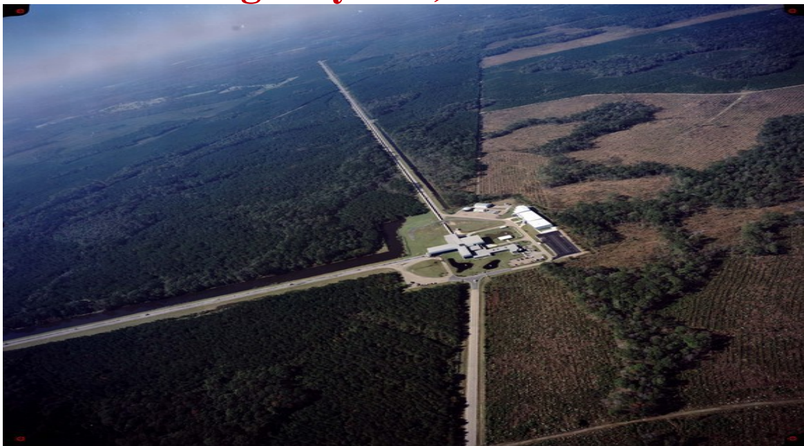
The LIGO facility in Livingston Parish, LA
